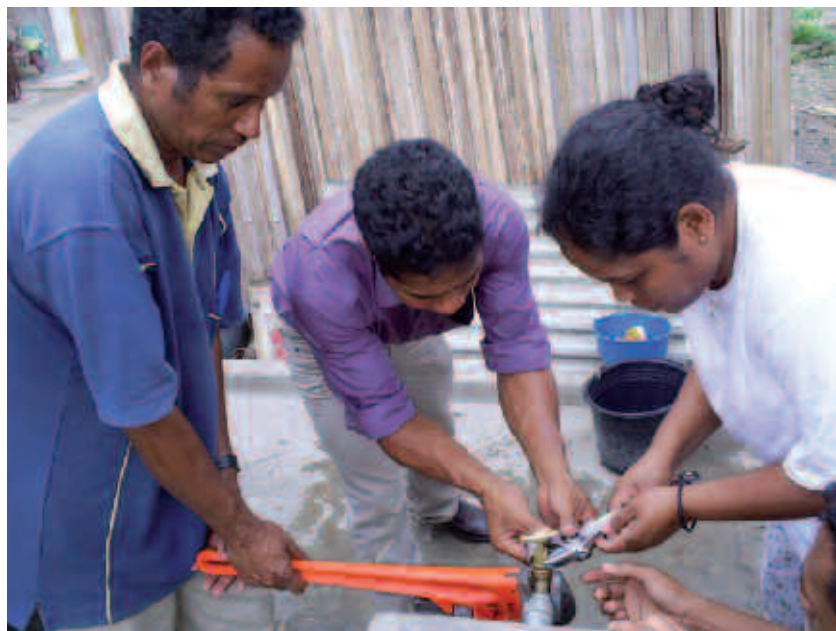
Practical training for members of the Water Management Committee: « How to repair a leaking tap? »
