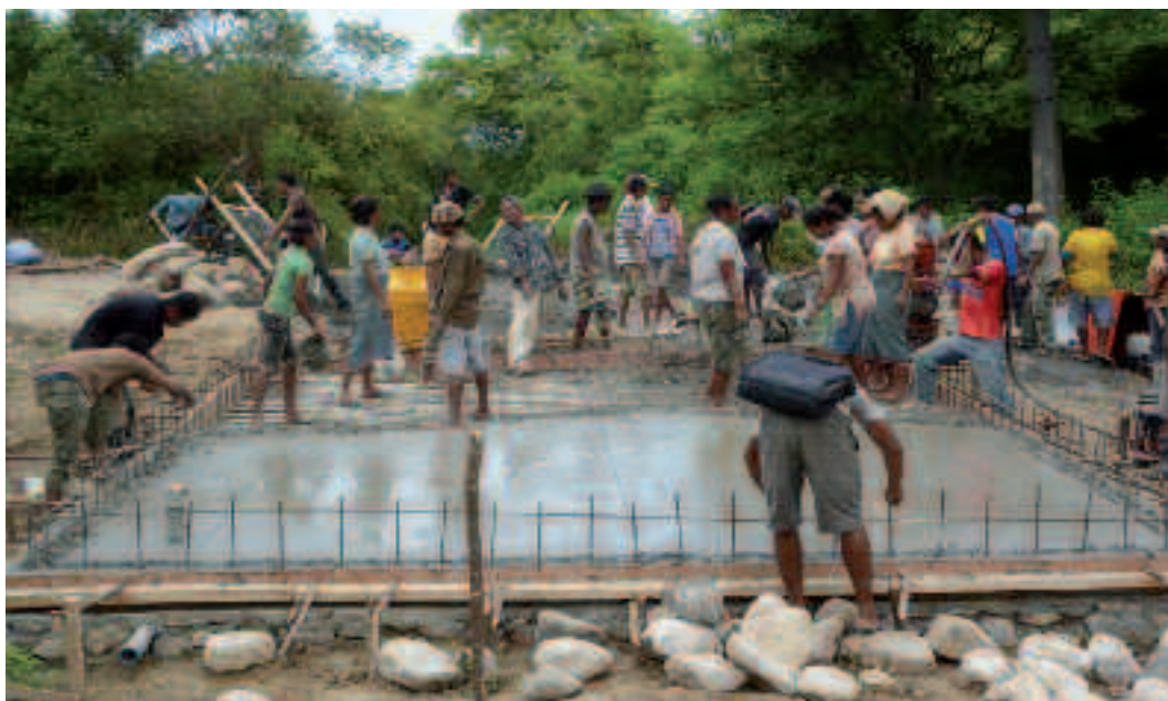
Construction of a water storage tank / Triangle G H
