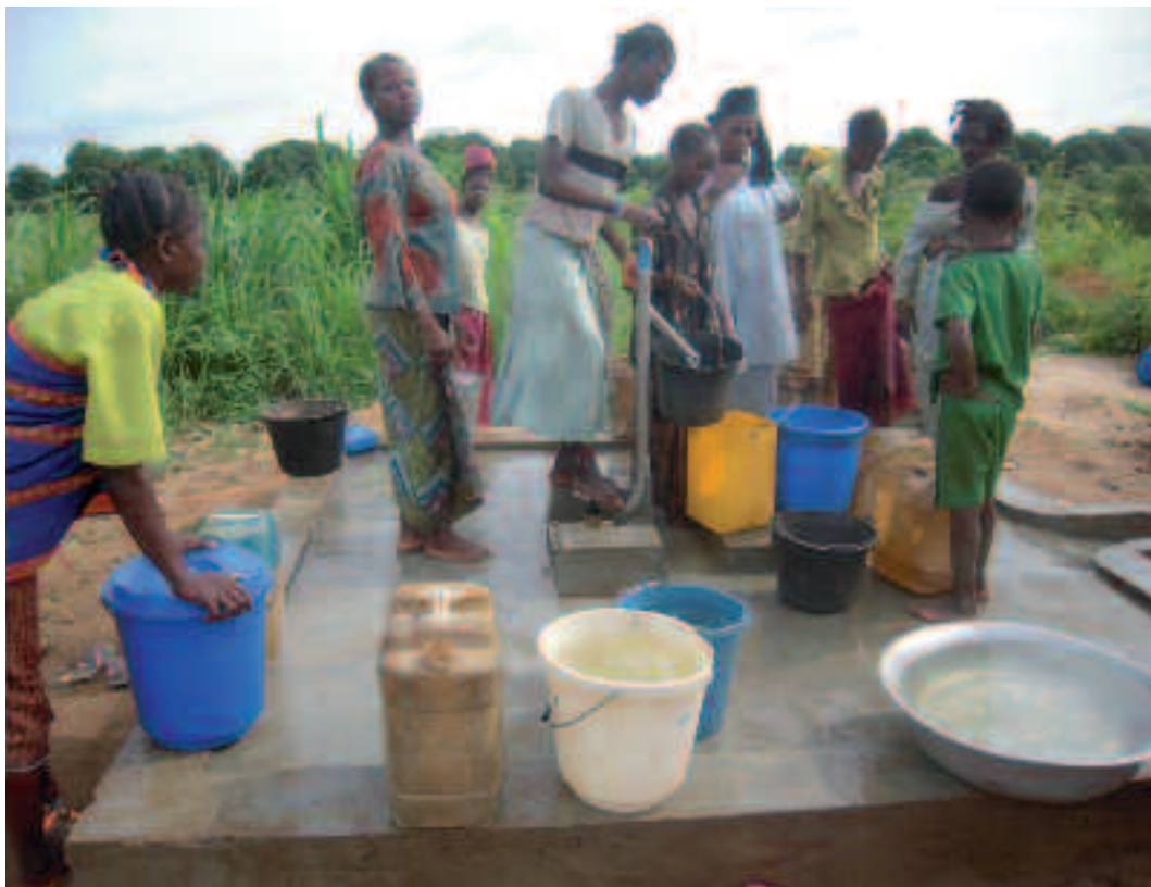
Borehole equipped with a foot pump in Sam Ouandja / Triangle G H
