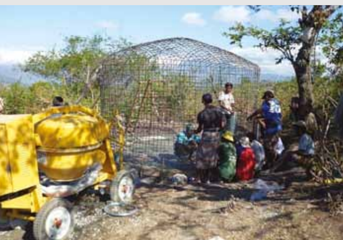
Installation of the metal framework for the construction of a ferrocement tank – Oecusse Province, East Timor
