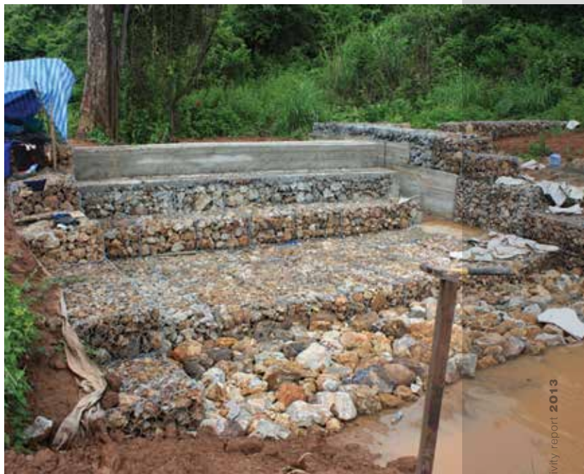
Laos – Bualapha – Gabion dam. Photo: Quentin Rouveïrolles / Triangle G H
