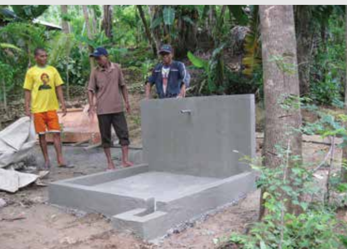
Timor Leste – District of Oecusse. Construction of a standpost. Photos: Francisco Suni / Triangle G H
