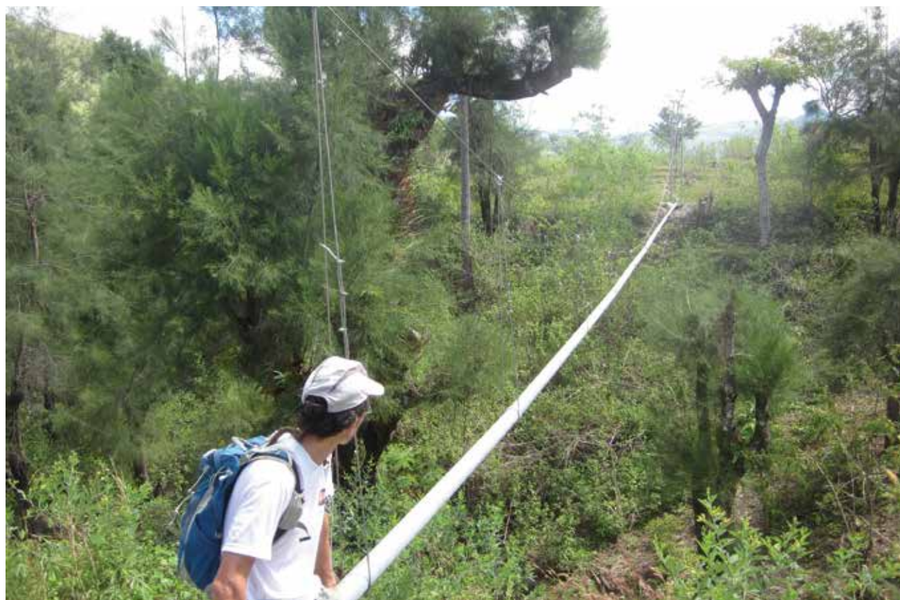
Timor Leste – Banafi – Construction of a suspension bridge to install a water line. Photo: Joël Terville / Triangle G H
