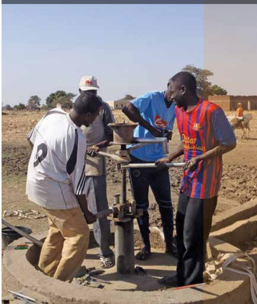
Sudan. Repair of a hand pump. Photo: local team / Triangle G H
