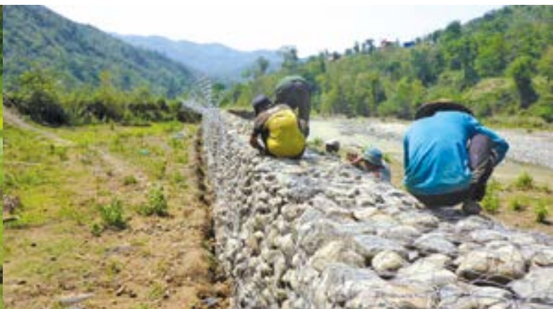
Installation of a gabion in Saru Plot, CawngThia Village, Burma. May 2018 ©Marc le Quentrec
