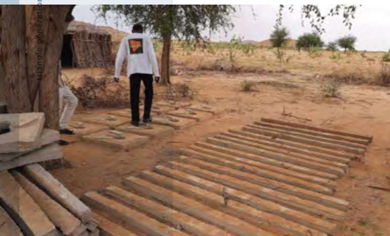
Construction of emergency latrines, Kreinik, Western Darfur, Sudan, © TGH
